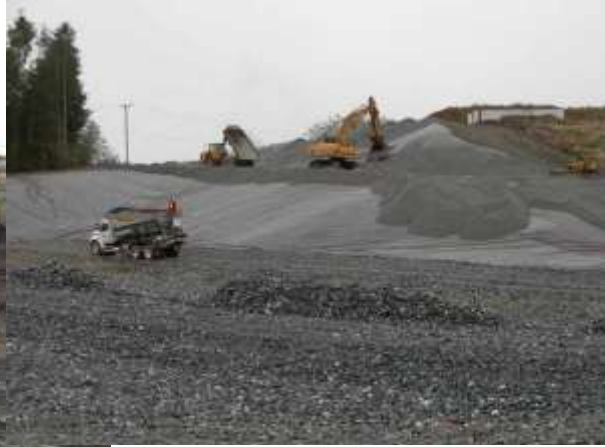
Photo 2: Phase 3 Expansion with Liner and Aggregate Cover
