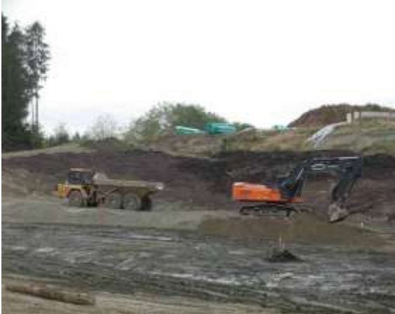
Photo 1: Phase 3 Expansion Excavation
