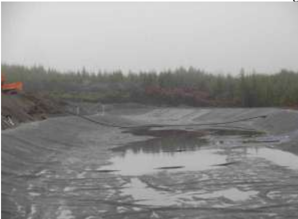
Photo 3: Equalization Pond with Liner
